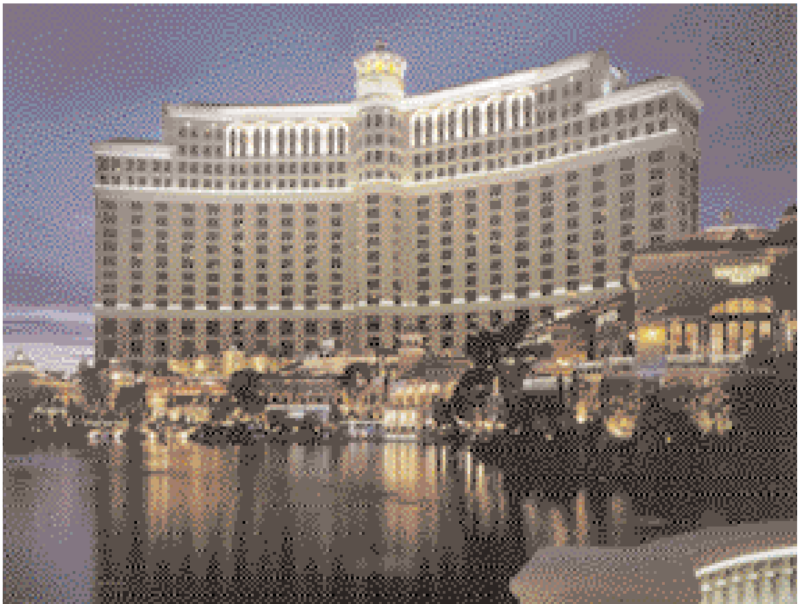
The Bellagio hotel and casino in Las Vegas shares more than 100 channels of music with its sister hotels, the Mirage and Treasure Island, through a networked fiber-optic audio system using
